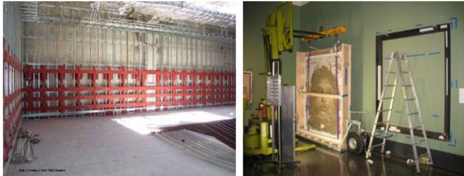
Figure 6. Installed behind the gallery walls of the Getty Museum at the Villa are a series of steel beams that are used to anchor large wall hung objects securely to the building, such as this large mosaic.
