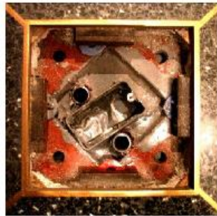
Figure 7. A floor anchor and an example of a pedestal anchored to the floor using the built in anchor points
